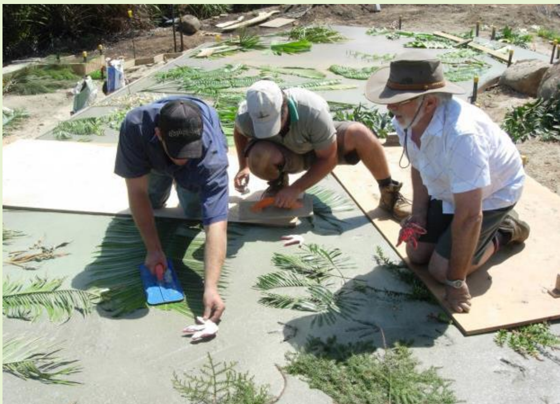
Lawrie Smith (right) making fossil concrete for the Coal Garden
