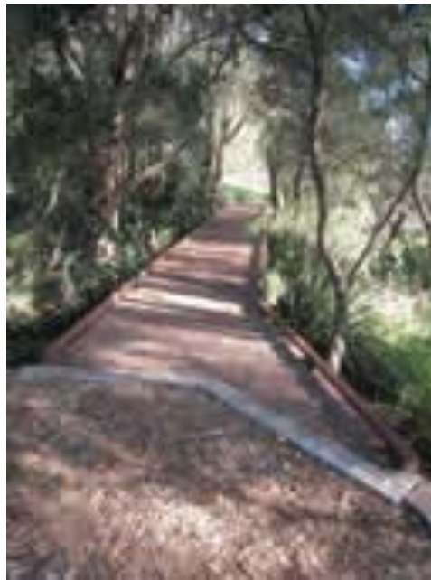
Newly constructed bridge across Butcher Bird Gully Photo: Paddy Lightfoot
